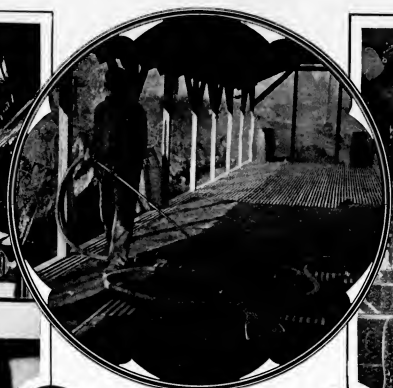
CLEANING CARPETS WITH COMPRESSED AIR UNDER 100-POUND PRESSURE AT THE MOTT HAVEN CLEANING YARDS OF THE PULLMAN COMPANY.
